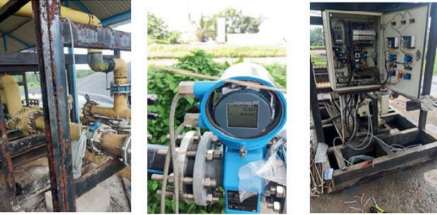
In this implementation, various instrumentation sensors such as Pressure, Flow, Temperature, and Flare status are integrated with Programmable Logic Control (PLC). The PLC acts as the system's brain, managing and processing data received from these sensors. Once the data is processed within the PLC, the results are then visualized through a Human Machine Interface (HMI). The HMI serves as the access point for operators or users to monitor and control the system directly.
